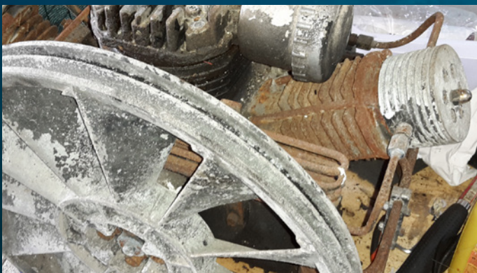
MCH 16 compressor before the service
